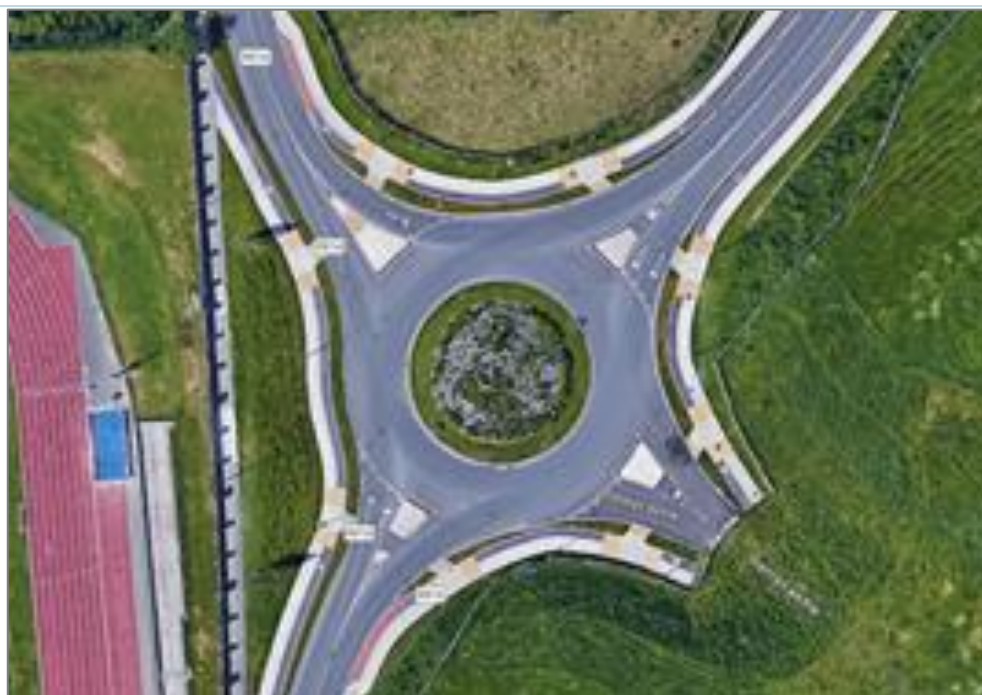
Figure 4-4 - Garrycastle Roundabout (Note: Fourth Arm has now been constructed connecting to IDA)
