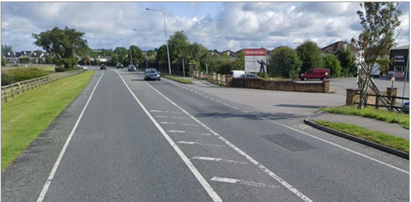
Figure 3-21 - Lack of Crossing Facilities and Tactile Paving
