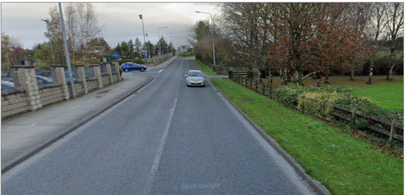
Figure 3-19 - Lack of Footpath Provision
