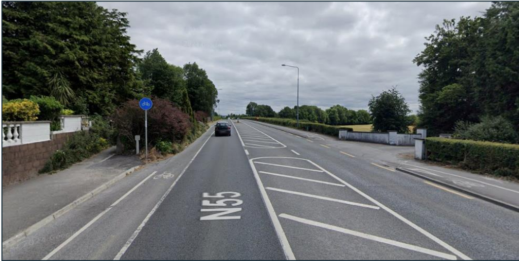
Figure 3-23 – Footpath Terminates (Left) w/ No Crossing Facilities Provided
